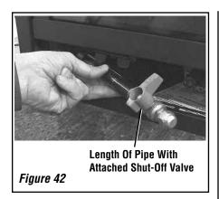
TEST ALL CONNECTIONS FOR GAS LEAKS (FACTORY AND FIELD):
